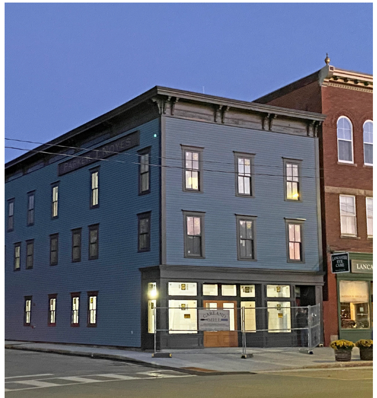
Redevelopment of the historic Parker J. Noyes building in Lancaster is nearly complete.
