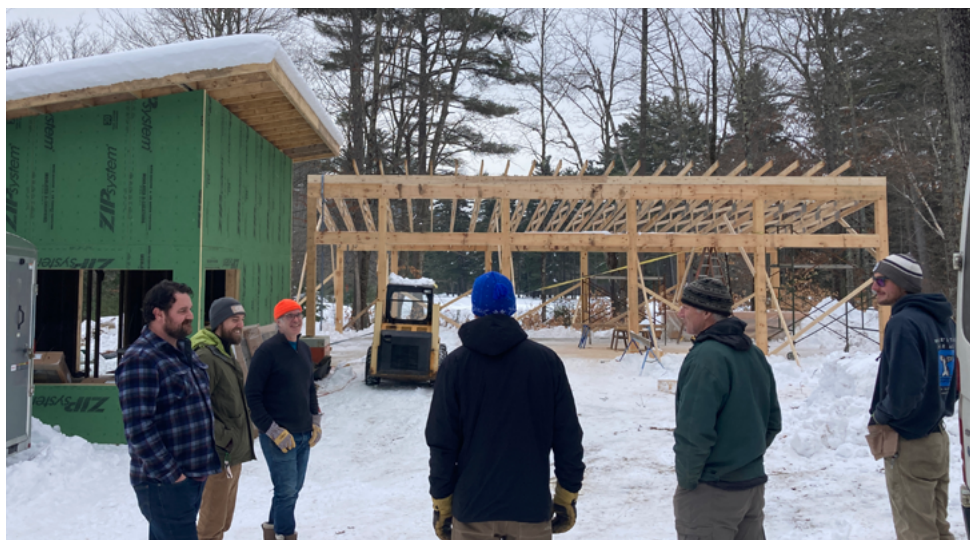
Construction of new trail center and pavilion.
