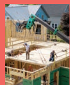
Cover photo: In Tupper Lake, N.Y., the Center is using mass timber and wood-based insulation in a new, nine-unit apartment building, supporting the forest products industry while creating new homes for residents and demonstrating the benefits of these innovative wood products. Photo by Rick Godin.
